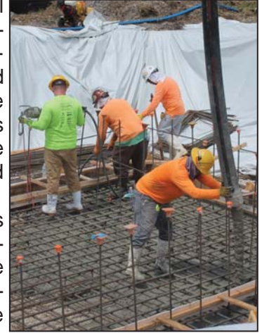
Pouring of concrete slab for new Brine Clearwell
