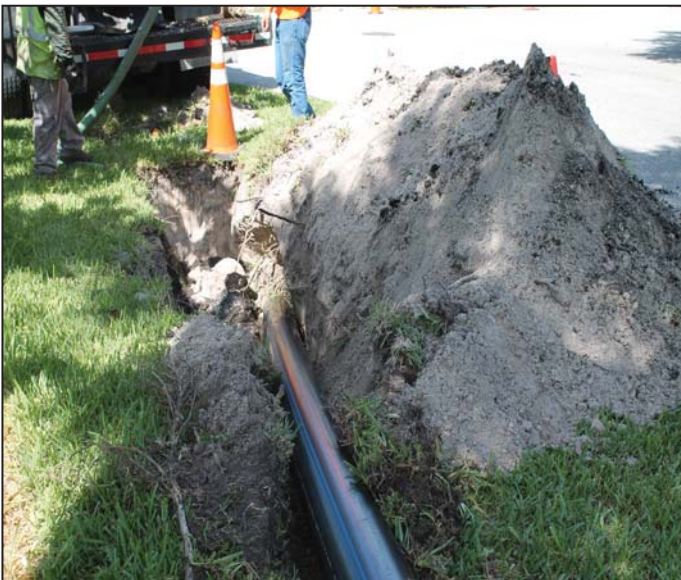
Directional bore with HDPE Pipe
