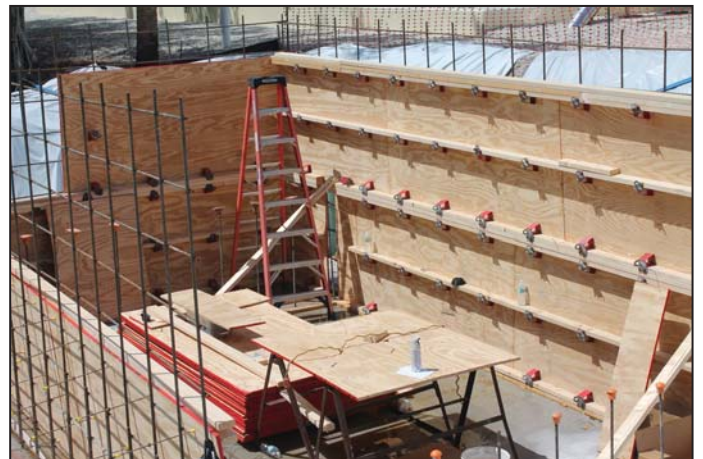
Framing the walls for the Brine Clearwell
