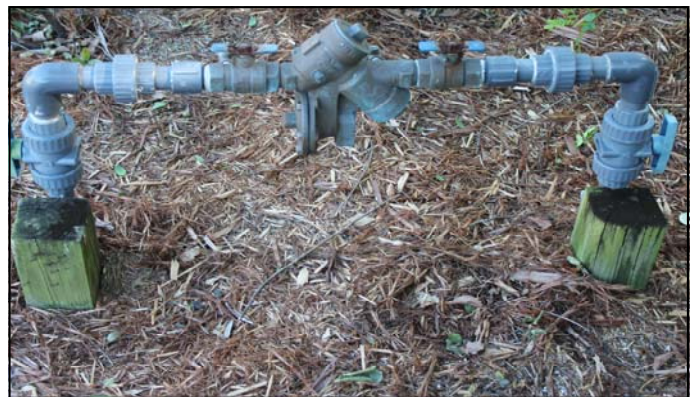
Reduced Pressure Zone Backflow Preventer
