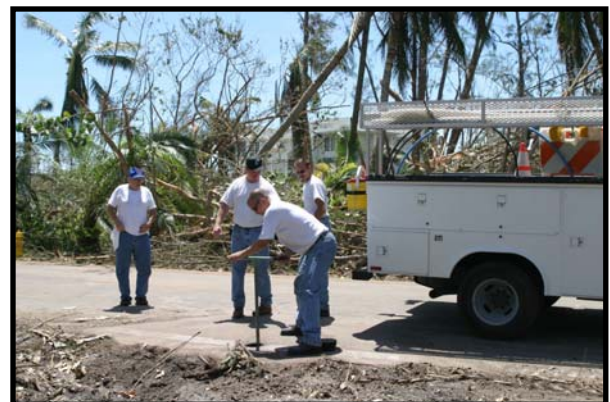
Brandon Henke checking a valve after Hurricane Charley.
