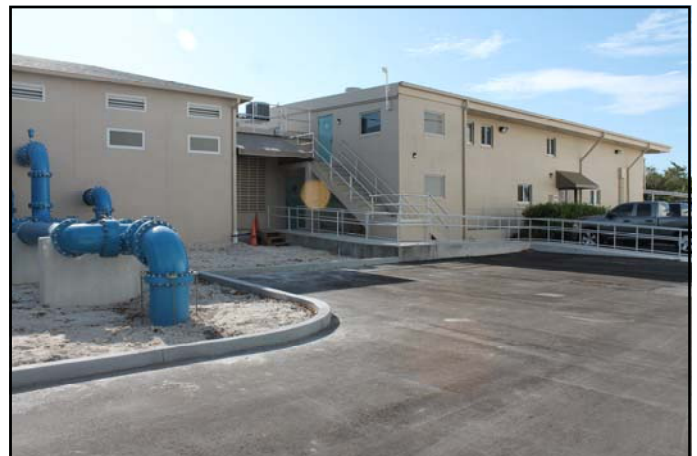
New High Service Building Curbing and Asphalt
