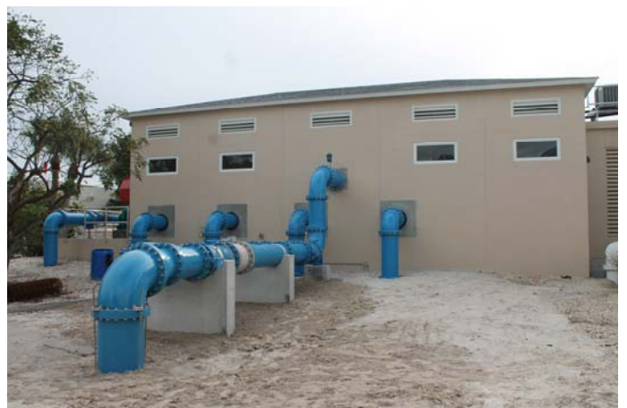
Exterior of new High Service Building
