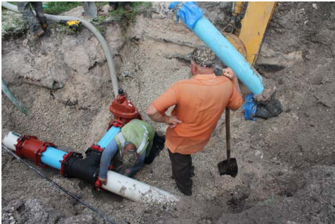
Making the connection from the old to the new system
