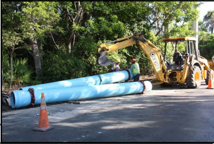
New 20" C-900 Pipe Staging
