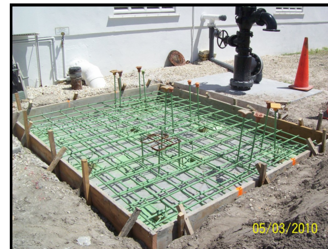
Concrete Header Slab
