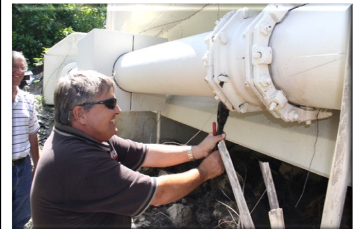
Ken Cabana Testing Stainless Bolt Galling on the Blind Pass Bridge Pipe Crossing
