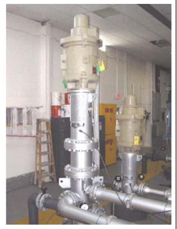
This new pump/turbine piece of machinery cost us around \$115,000, but we anticipate that it will save us around \$15,000 to \$20,000 per year in electricity! As one measure of the savings, the amperage required to feed water to RO Train B used
