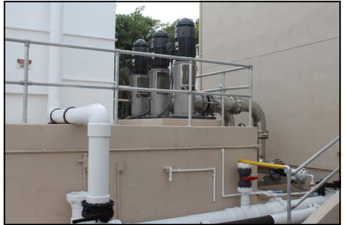
Current Product Clearwell, with Three Vertical Turbine Pumps and Motors Installed, as the New Brine Clearwell will have
