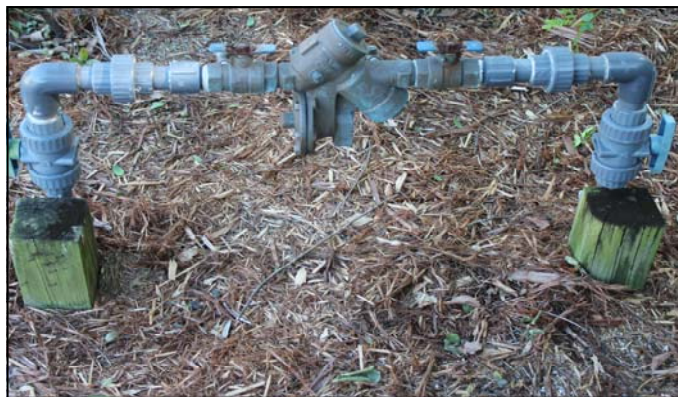
Reduced Pressure Zone Backflow Preventer
