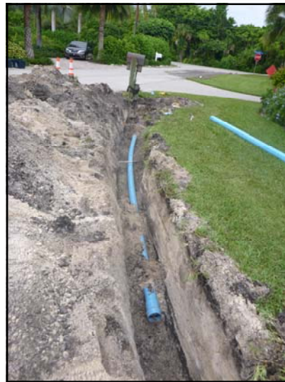
New Piping in Shell Harbor
