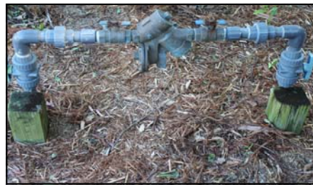
Reduced Pressure Zone Backflow Preventer
