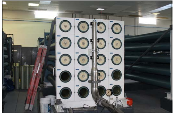
E Train Membranes Installed
