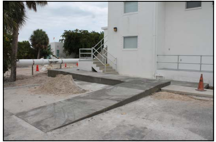
Replaced RO Plant Handicap Ramp
