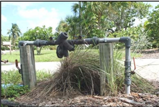
“Reduced Pressure Zone” Backflow Preventer
