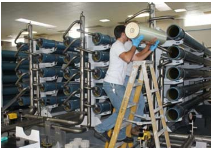
Membrane element being installed in a train vessel
