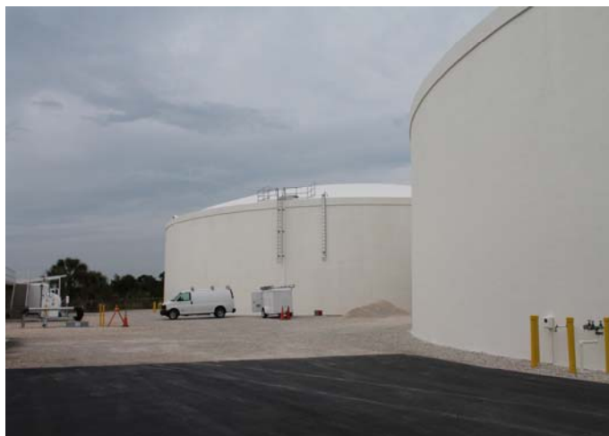
Newly cleaned and painted 5MG Storage Tanks
