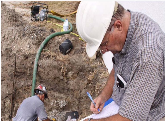
Jim Elliott & Corrosion Expert Examining Pipe
