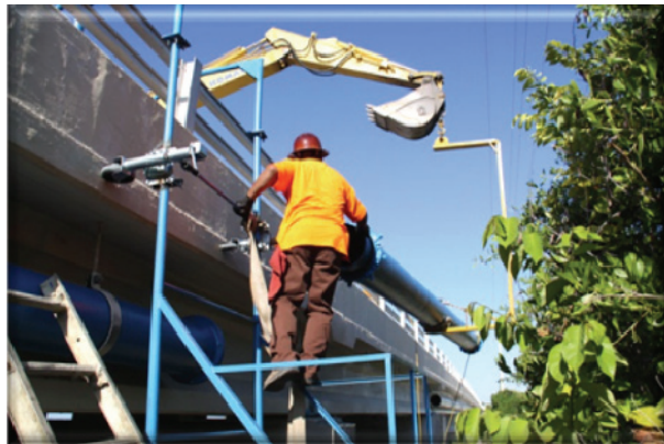
Blind Pass Bridge Pipe Work
