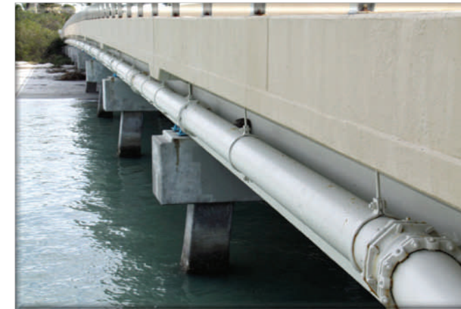
Blind Pass Pipe Replacement Project
