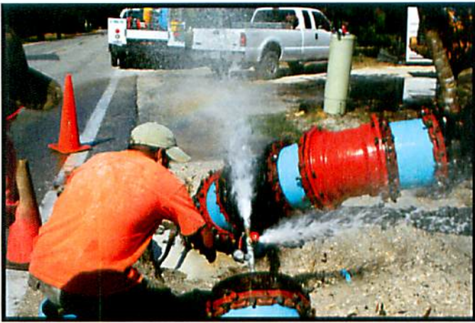
Preparation for testing the Line
