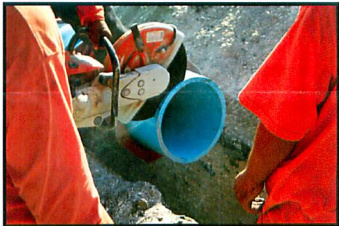
The Last Joint of Pipe is "Cut-to-Fit"
