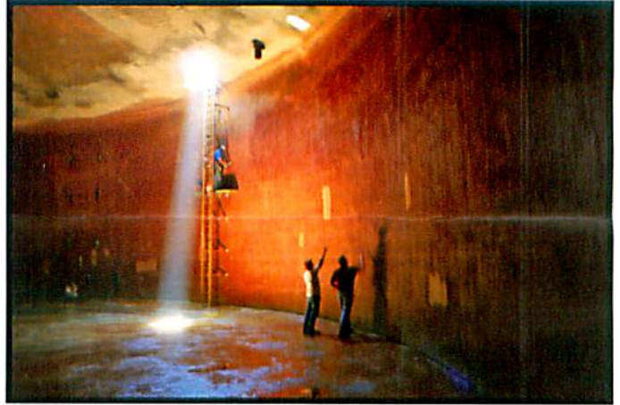
Internal Inspection of the two million gallon Periwinkle water storage tank
